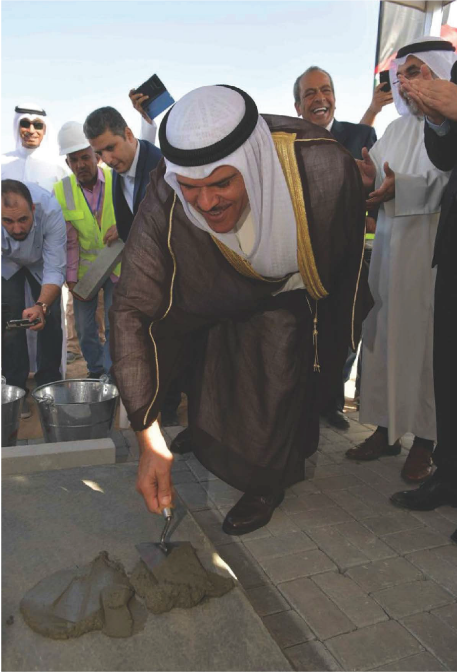
H.E. Sheikh Salman Sabah Al-Salem Al-Humoud Al-Sabah, Former President of Civil Aviation, laying the cornerstone of the new Control Tower on 23/11/2017.
